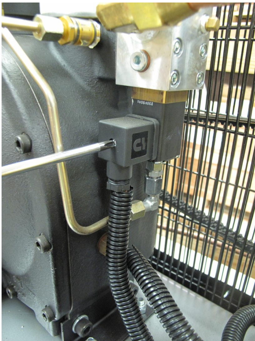
Install new solenoid
